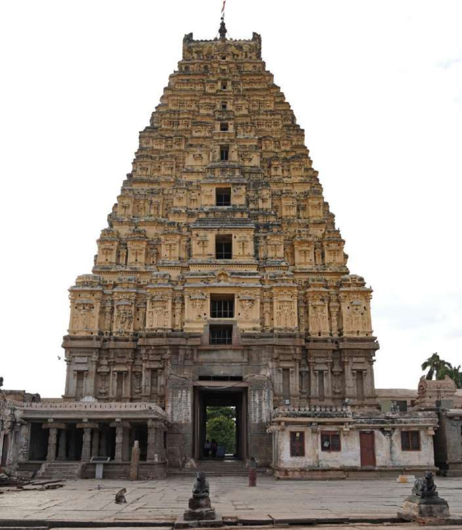
Main gopura and other structures on the east side
