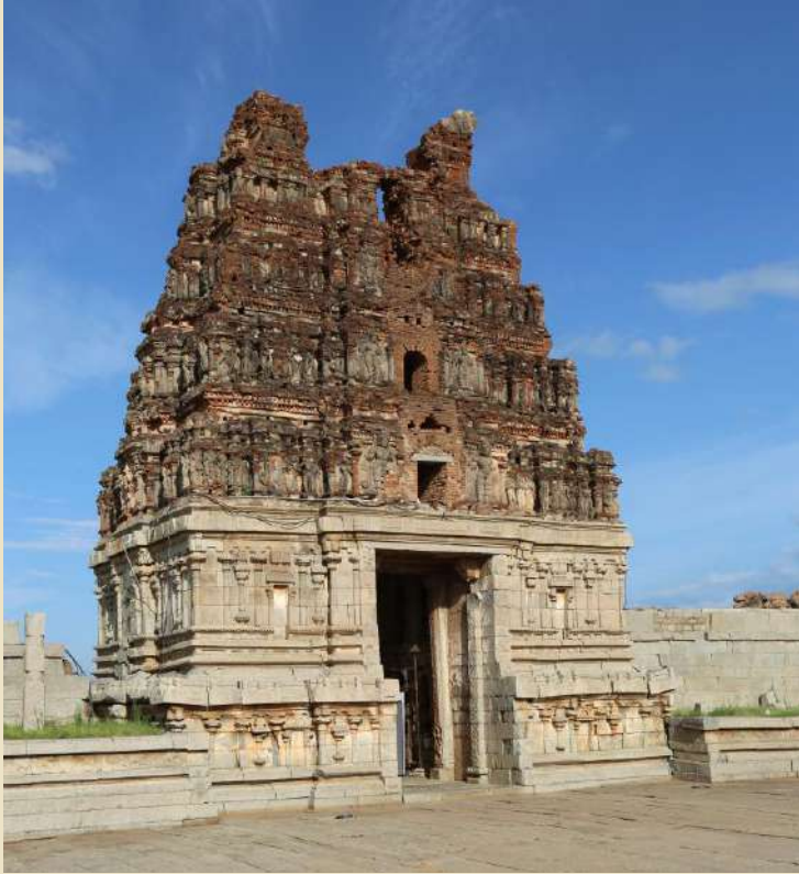
East Gopura (view from west)
